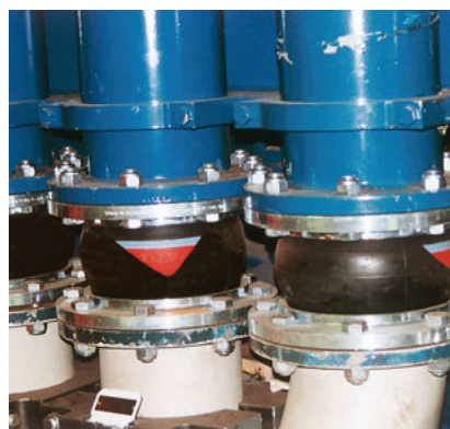
STENFLEX® Type RS-1 used in cooling water system of ship's engine
