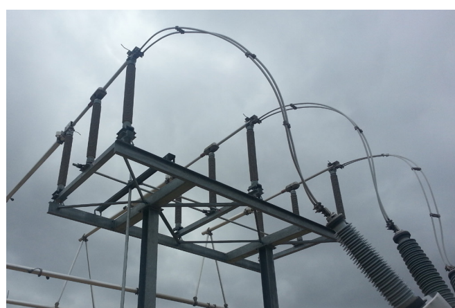
Simple Construction: the blade is the current path, no complex hinge transfer points.
