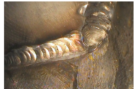
Weld of a Heat Exchanger Tube
