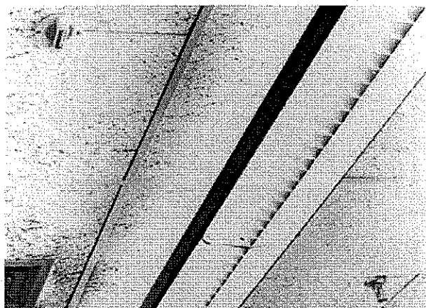
FIGURE 5: Typical ceiling installation of a horizontal DETECT-A-FIRE model. Here it is used in combination with a sprinkler system to detect overheat and actuate an alarm.
